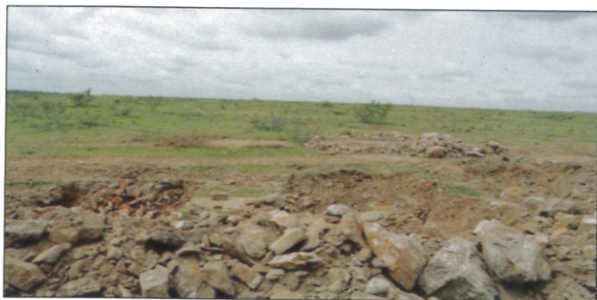
Fig. 3. Panoramic view of side slopes, shoulder slopes and backslopes on the eastern side of the site
