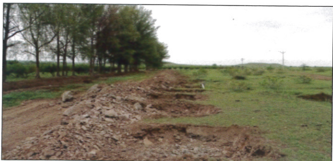
Fig.2. Exposure of rock outcrops on the backslopes of western side
