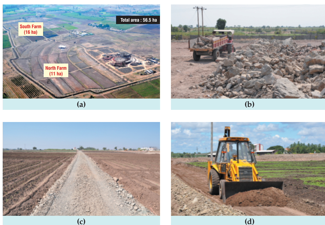
Fig. 1.4. Aerial view of the farm (a), Farm road development: heavy stones as bottom layer (b), murrum as top layer (c) and roads after completion of work (d)
