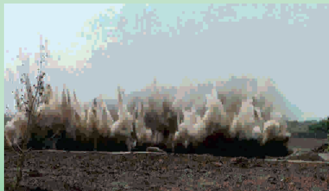
Blasting of hard pans
