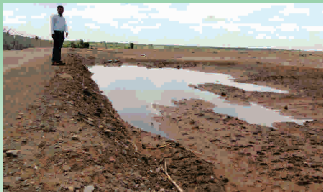
Water harvesting on laying peripheral roads
